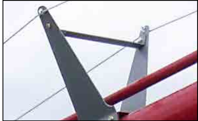
Fig 40 - Cable clamps on truss risers
